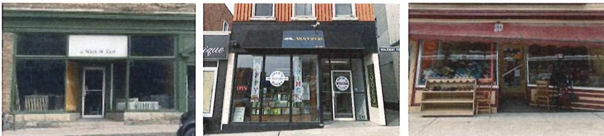
Plate 5 Examples of storefronts within the HCD.
