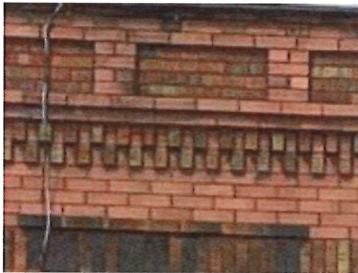
Colour difference due to accumulation of dirt on brick. Cleaning for aesthetics reasons may be considered.
