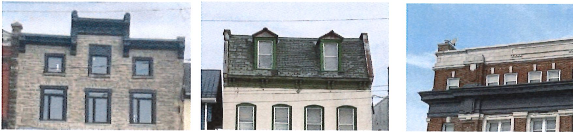
Plate 8 Examples of parapets and roof types in the commercial corridor of the HCD.
