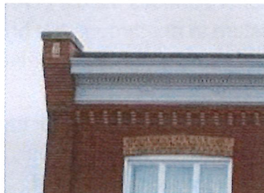
Elaborate brick detailing should be preserved.
