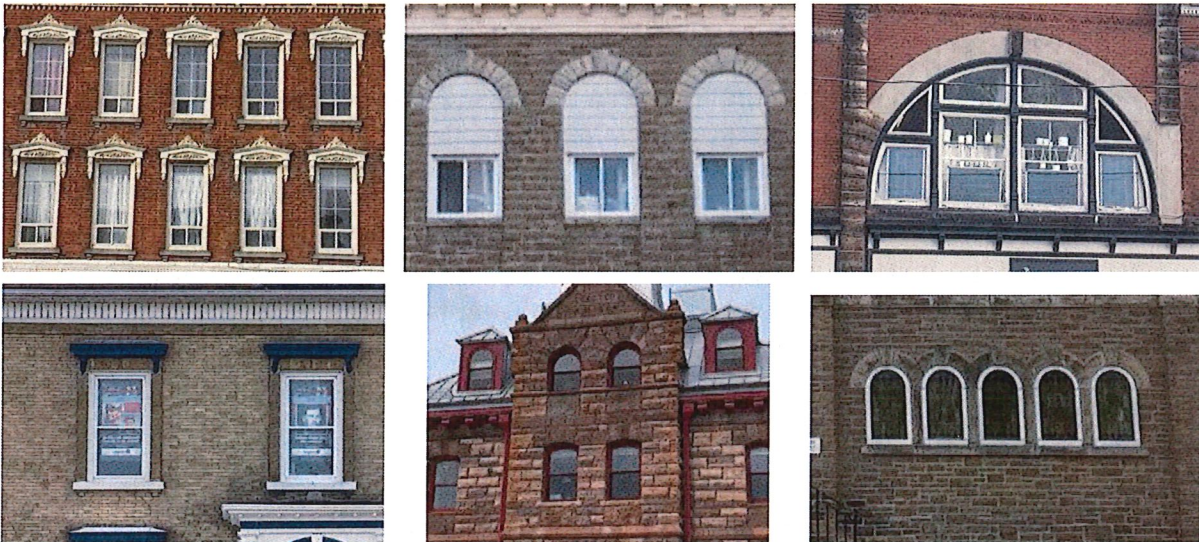
Plate 4 Examples of window types and shapes in the HCD. Rectangular, round arch and segmental arch are most common. Avoid incompatible infill in historic windows (example in top middle photo).
