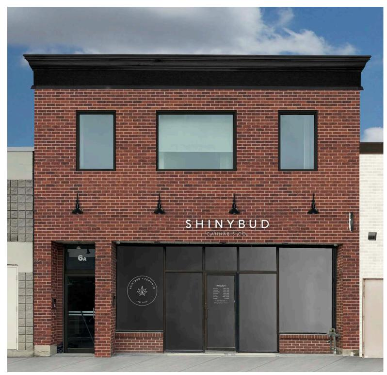
ADDITIONAL NOTES: 1) EVALUATE BRICK ONCE EXISTING SIGNAGE IS REMOVED. 2) ADD J-BOXES FOR GOOSENECK LAMPS. 3) PAINT EXISTING STOREFRONT DOOR TO APARTMENTS TO MATCH.
