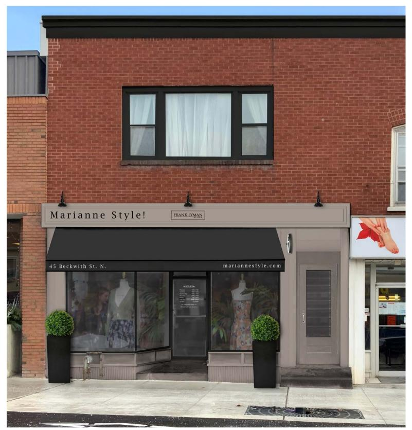
ADDITIONAL NOTES: 1) REMOVE ACRYLIC SIGN / AWNING. 2) REPLACED DOOR TO APARTMENT SHOWN. 3) ADD J-BOXES FOR NEW GOOSE LAMPS
