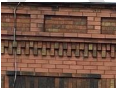
Colour difference due to accumulation of dirt on brick. Cleaning for aesthetics reasons may be considered.
