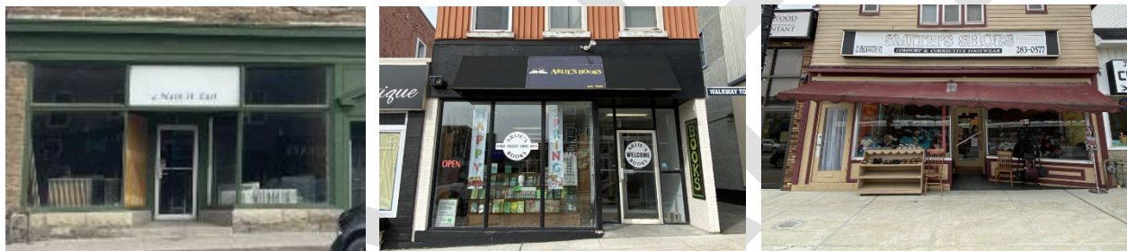
Plate 5: Examples of storefronts within the HCD.
